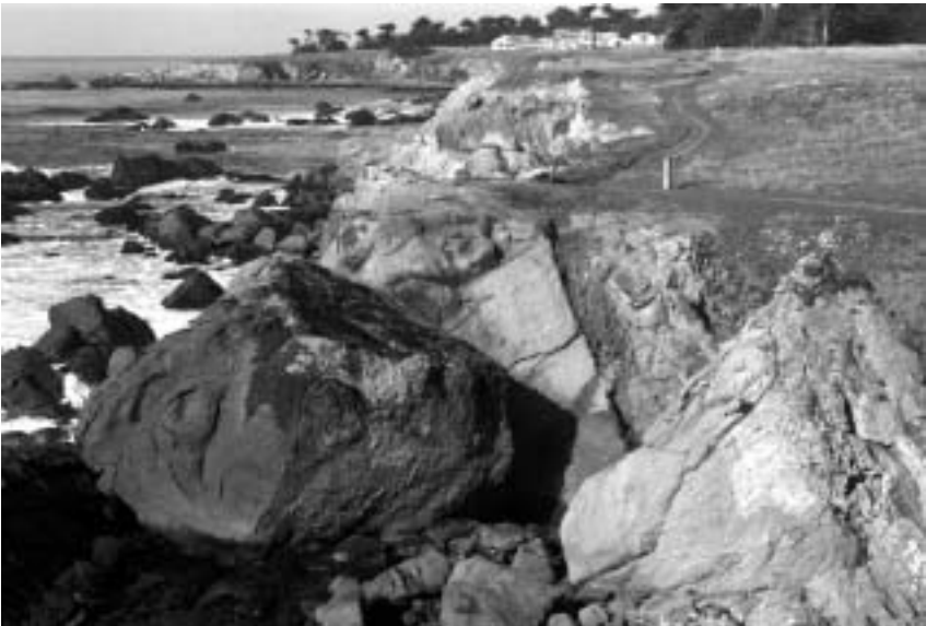
A large block of sandstone has broken from the bluff near Tide Pool and is now in the surf zone being broken into smaller pieces by wave action.
